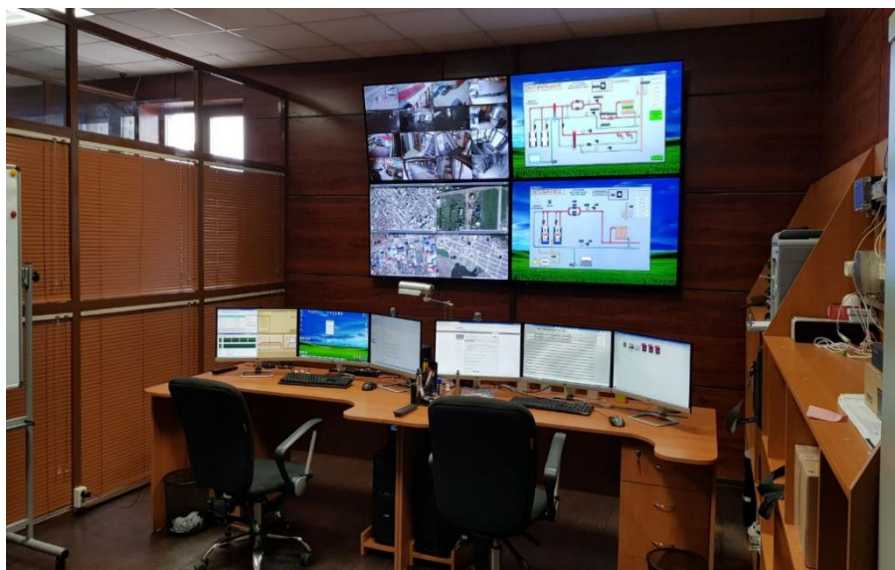
Fig. 4. Dispatching office of LLC "Energoberegayushchiye Tekhnologii" for remote control of energy consumption systems
